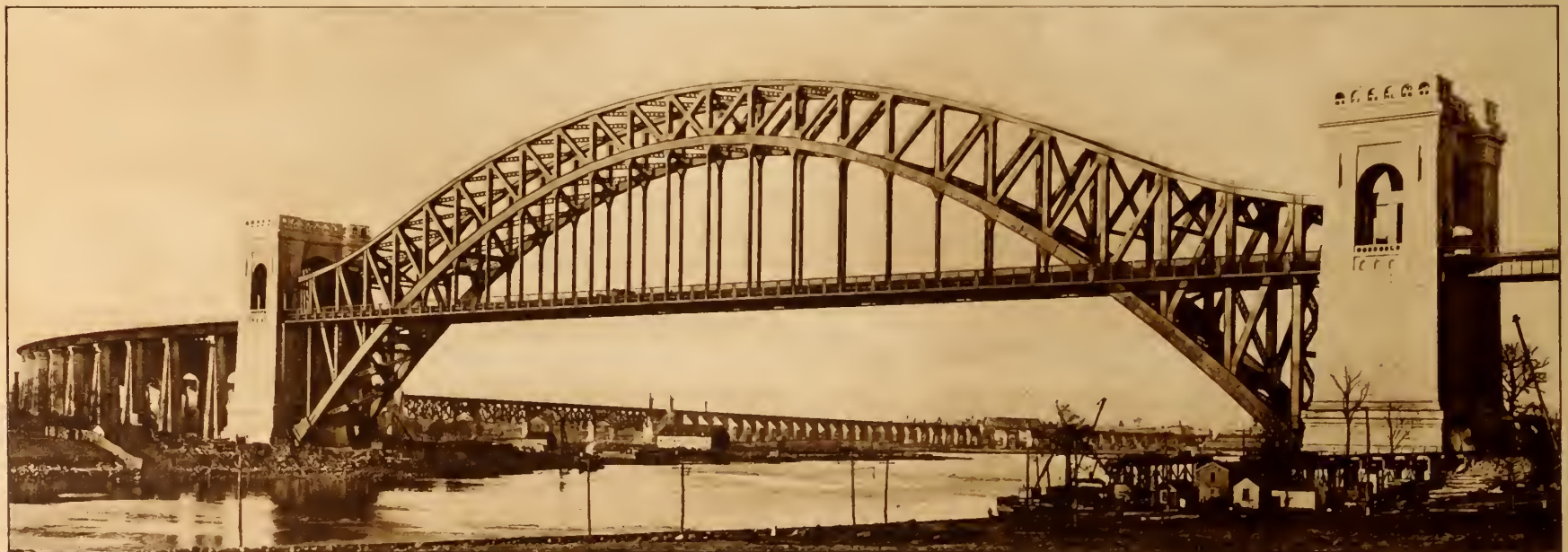
HELL GATE BRIDGE, connecting Pennsylvania Railroad trains in Brooklyn to the New Haven trains. One of the largest bridges in the world, extending a thousand feet in length. © Irving Underhill
